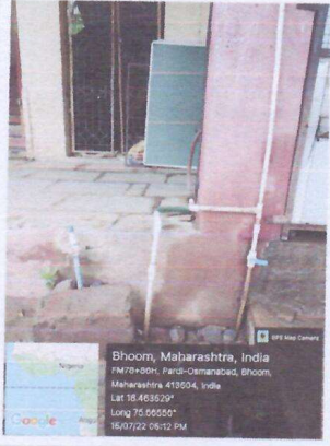
WATER DISTRIBUTION SYSTEM IN THE CAMPUS
